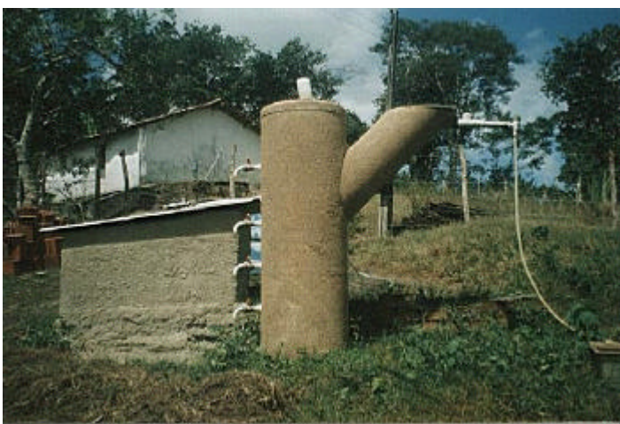
FIGURA 3. Reator UASB
